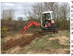
The driveway next to the scrutineering area with its potholes is compressed sand, quite different to the driveway from the road to the car park. It was decided to remove the ridge between the tracks using this and other material to fill the potholes. This are was then cordoned off to give it time to drain before traffic is allowed to use it again.
